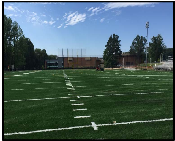
Figure 1: A synthetic turf field under construction (USEPA, 2016a)
