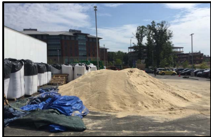
Figure 4: Sand and packaged crumb rubber awaiting field installation (USEPA, 2016b)
